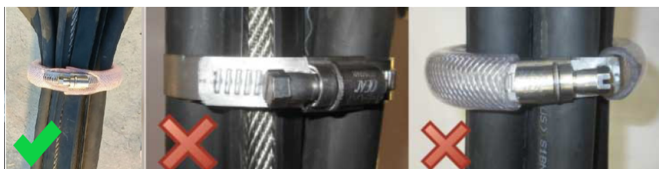
Fig. 19: Installation information for the cable clamps
